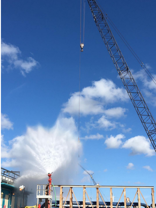
Photo from the Port of Corpus Christi Authority Avery Dock drill, posted to the LEPC Facebook page - The LEPC participated as a drill observer
